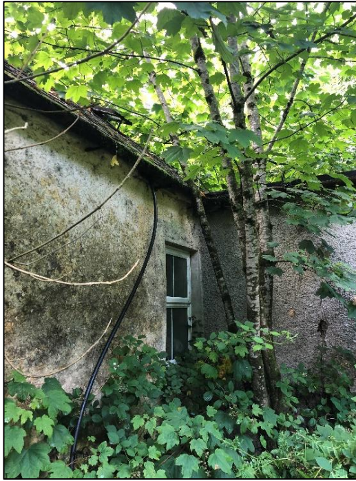
Plate 4-3 Back of derelict dwelling with large gaps along fascia.
