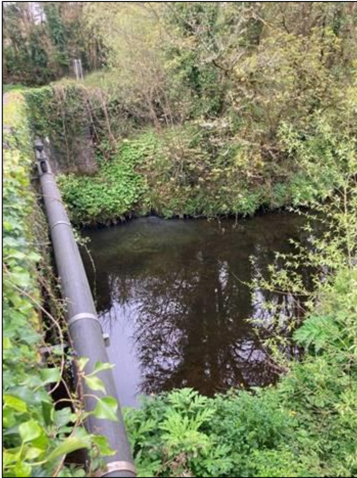
Plate 5-1 Bridge 1 existing ducted services.
